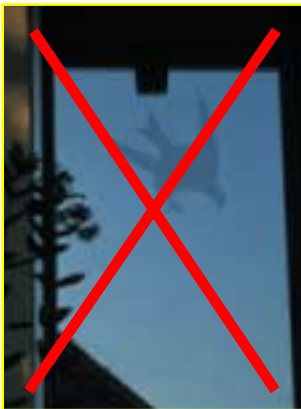
Not suitable: Black bird silhouettes are often hardly visible and are not effective.
