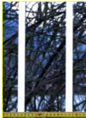
For home use: Vertical strips of insulating tape and non-reflective adhesive tape (e.g. Scotch Magic 810) offer good protection but do not last very long.
