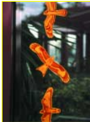
Only partly suitable: Coloured raptor silhouettes offer some protection. Several silhouettes should be applied per window pane.
